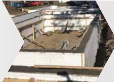
Fox Blocks reinforced concrete walls inevitably last forever. The EPS insulation does not deteriorate, absorb moisture or promote mold or mildew. The pool wall assembly will be able to withstand weather and everyday lifestyle events. The solid wall assembly does not expand and contract like a metal pool wall assembly, providing a more stable substrate for the pool finishes.
