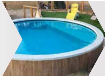
The simplicity of Fox Blocks as a modular produce does allow for a do-it-yourself application. The footings and pool walls must be designed to accommodate the loads on the wall from the water and the earth. The footing and wall assembly will require reinforcement bars installed as per design specifications. This picture is of an award winning DIY Fox Blocks pool.
