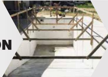
Fox Blocks are 16" x 48" providing 5.33 sq.ft of wall area per block. Installation is very easy and depending on the overall pool layout and design complexity, the blocks for the pool walls and the concrete placement should be able to be installed in one or two days.
