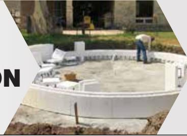
Solid monolithic reinforced concrete provides a high structural capacity for below grade and/or above grade walls, any height, any overall size. Modular ICFs provide a continuously insulated wall with a solid substrate for any pool finish. The base footing and concrete walls must be designed to suit the structural requirements.
